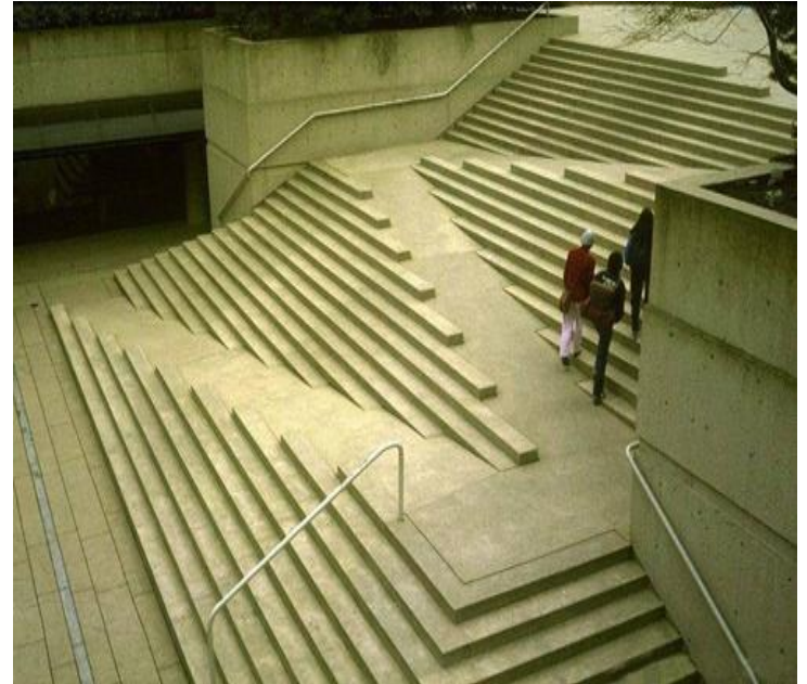
Stair/ramp designed by Cornelia Oberlander and Arthur Erikson in Robson Square, Vancouver
